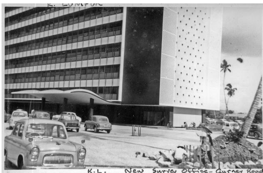
K.L. New Survey Office - Gurney Road
