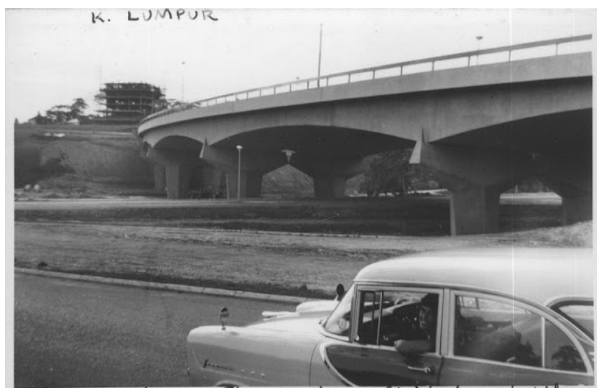
Flyover to unfinished Parliament Building, Kuala Lumpur
