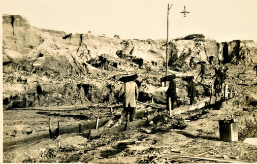
Open Cast Tin Mine.
